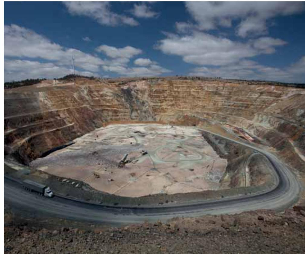
Set up in a disused zinc mine, the bioreactor "digests" 500,000 metric tons/year of household waste from the Sydney agglomeration.
